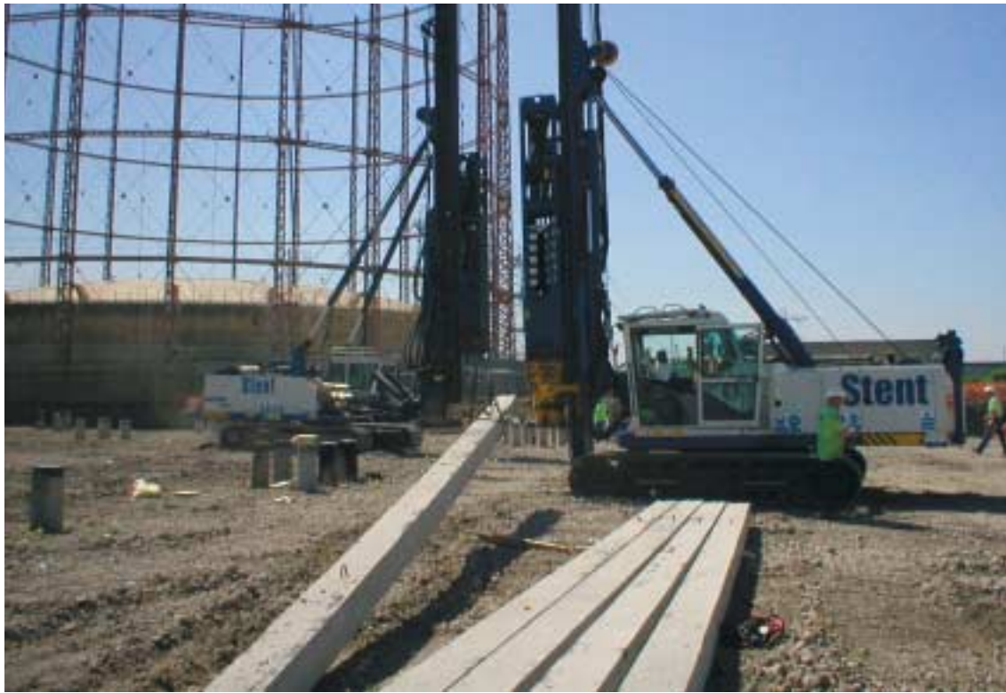
Supports being laid at the new IKEA site in Edmonton 19/5/04
